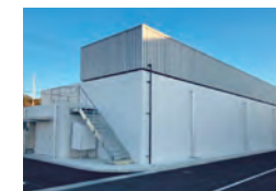
Wastewater treatment tank
