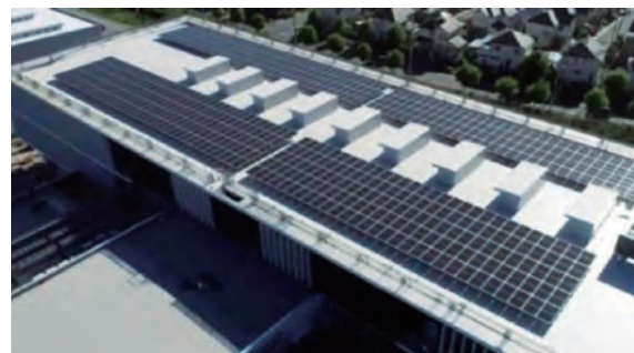
Solar power generation panels that have been installed over the entire roof of the Kobe Science Park Center office building
